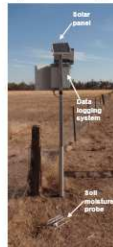
Fig. 4. Set up of a typical semi-permanent station
